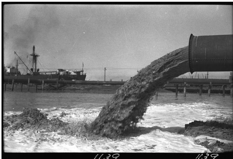
1139 No. 1 Appleton Dock. Discharge from suction dredge 'G.F. H.' into reclamation basin. (Public Records Office Victoria).
